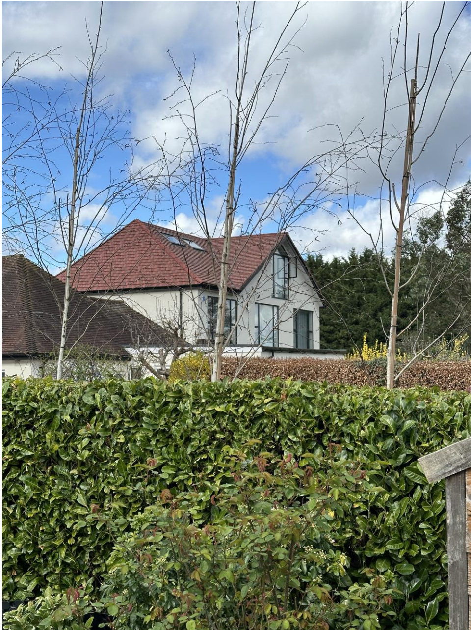
Figure 22 – Photo of Hillyfields (No.11 Hayes Mead Road)
